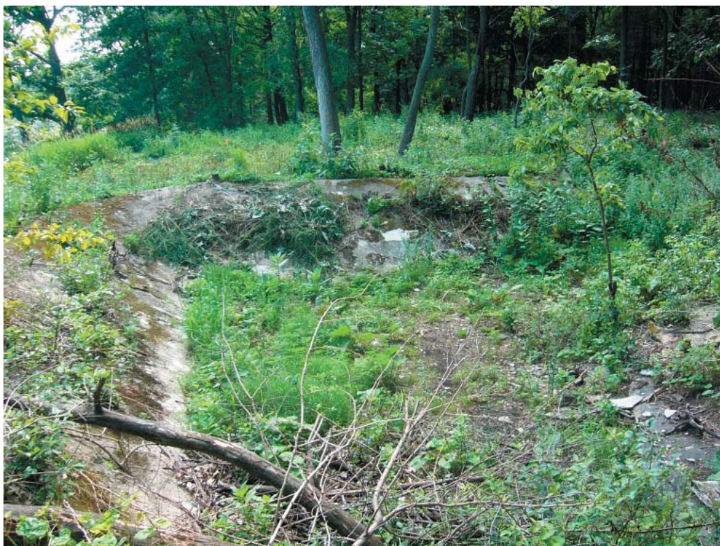
Upper cistern of waterfall system, view to southwest.
