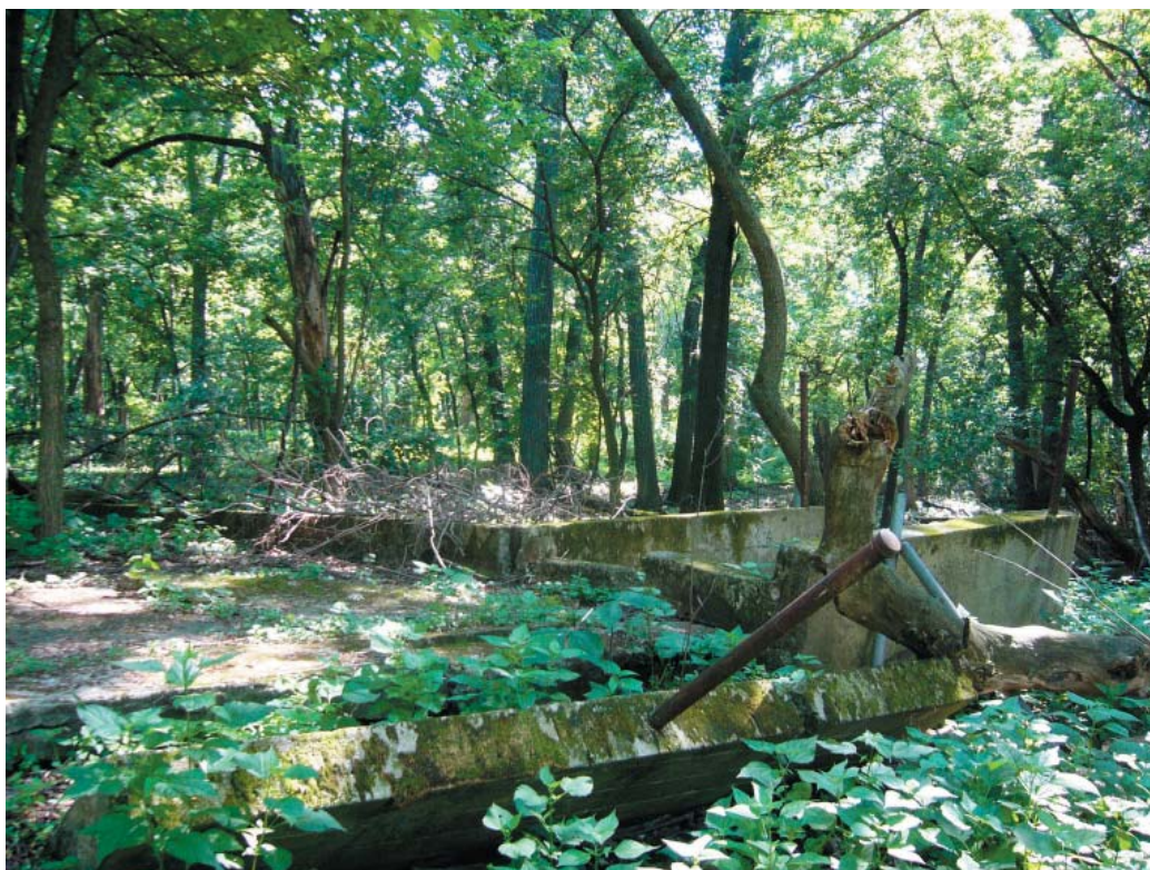
Hog barn, view to southwest.
