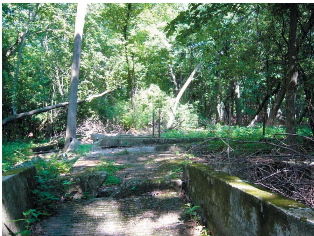
Hog barn, view to the west.
