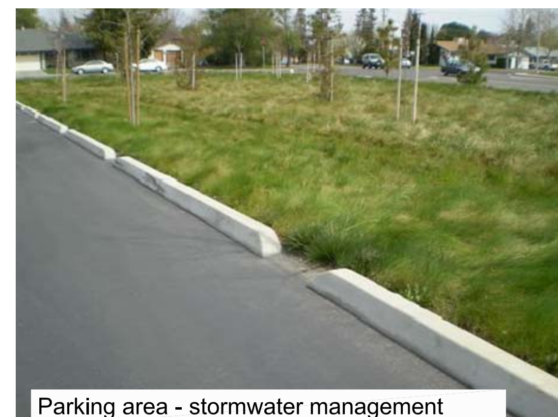
Parking area - stormwater management
